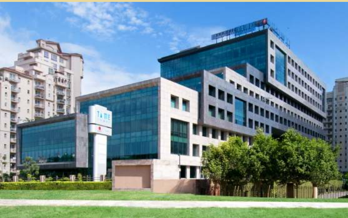
Time Tower, Gurgaon 7 Star Office Complex
